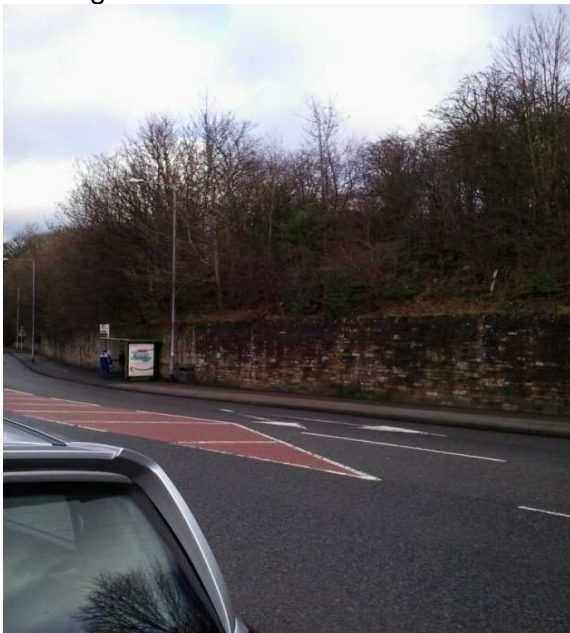
Figure 5 showing height of wall plus banking behind (note relative size of bus shelter)
